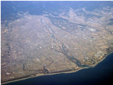
Figure 2 Tenryu River near Hamamatsu City, Shizuoka Prefecture
