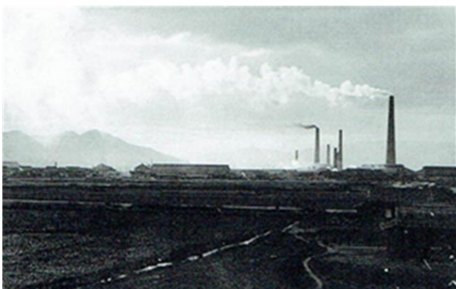
Photo 4 The actual state of smoke injury
