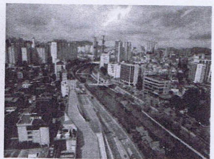
Fig.14 Elevated highway and a covered road were removed, and a blue sky appeared.
