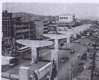
Fig.10 The supporting beams of the elevated highway
