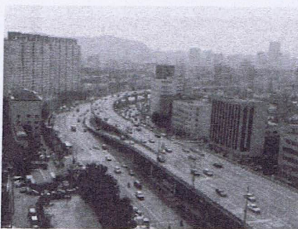
Fig.12 Lump of concrete running over a river
