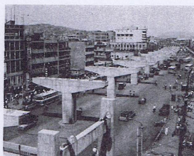
Fig.10 The supporting beams of the elevated highway
