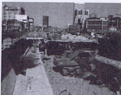
Fig.13 Construction for reproduction
