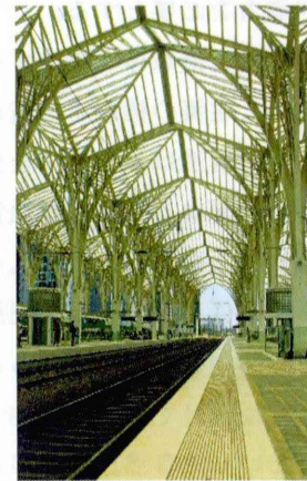
(c) Oriente Station
