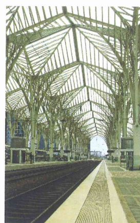
(c) Oriente Station
